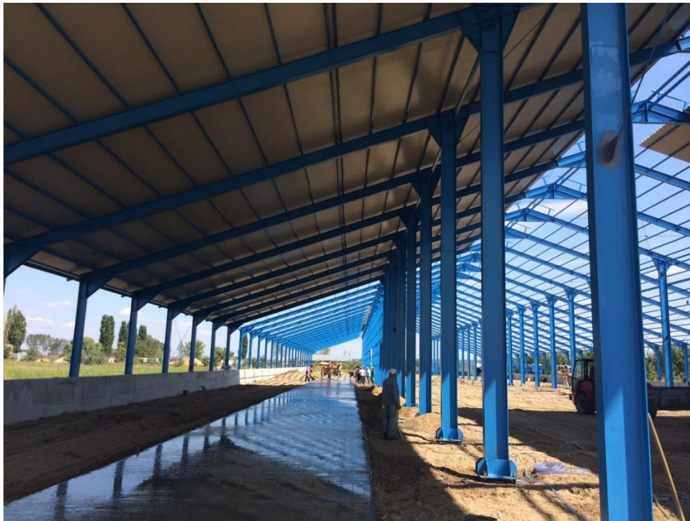
BETONARE ALEE RACLOR
